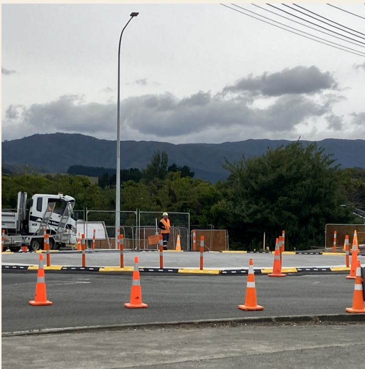
Mill Road / Rahui Road roundabout
