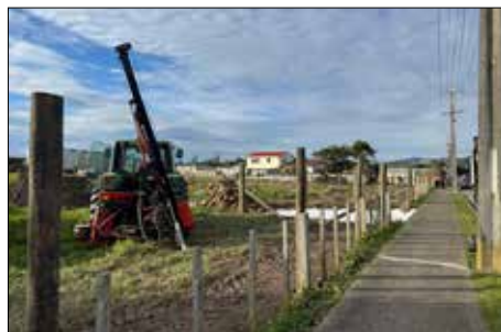
Work under way at the Rangiorua Road development. Photo supplied
