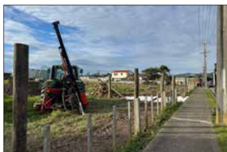
Work under way at the Rangiorua Road development.
