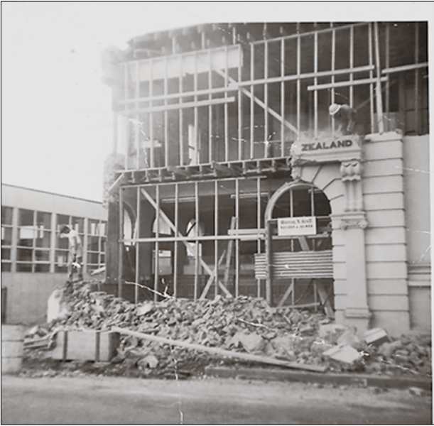
The façade of the BNZ building being demolished in 1966.
